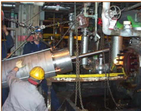
Rotor Installation
