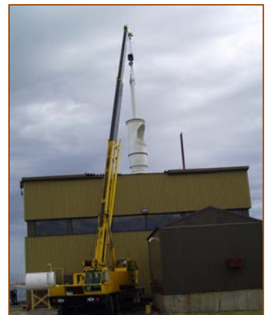
Installing Repaired Circulating Water Pump
