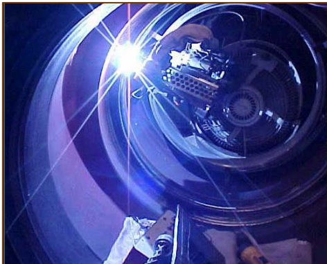
Feed Pump Barrel Weld Repair
