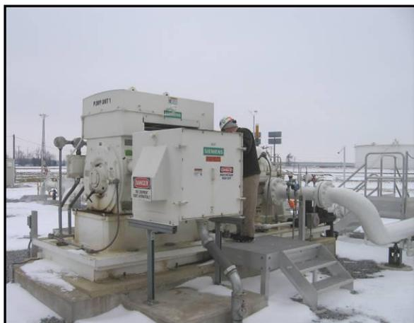
**Figure 5 – Main Line Pumping Unit (MLPU)
