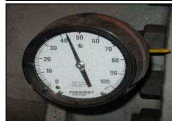
**FIGURE 20: SUCTION (TOP) AND DISCHARGE (BOTTOM) PRESSURE GAGES TYPICAL FOR ALL PUMPS**
