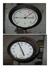
FIGURE 20: SUCTION (TOP) AND DISCHARGE (BOTTOM) PRESSURE GAGES TYPICAL FOR ALL PUMPS
