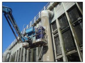
FIGURE 3: FLOW METERING ON RISER #7
